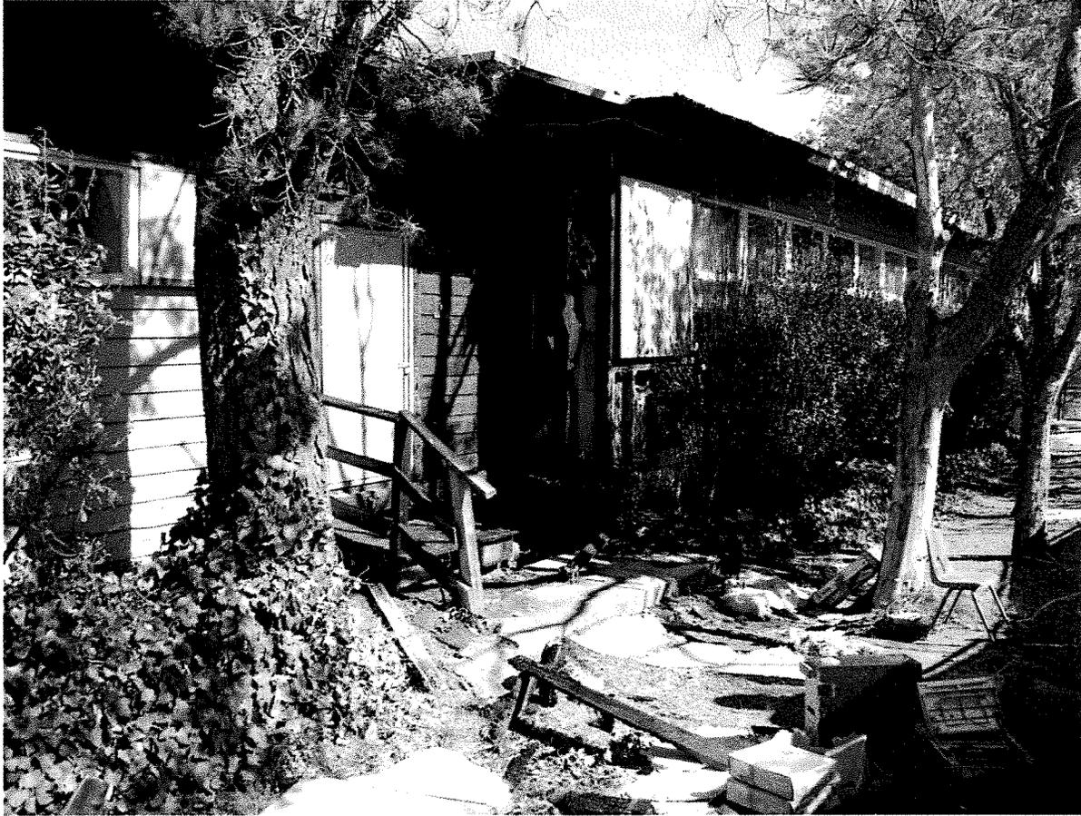
From the exterior, there is surprising little indication of the fire from the south, east and west sides, but on the north side (up the hill), the entry patio has collapsed due to burn damage, several of the foundation wood panels have burned out, and smoke and fire damage on the building exterior is evident.
