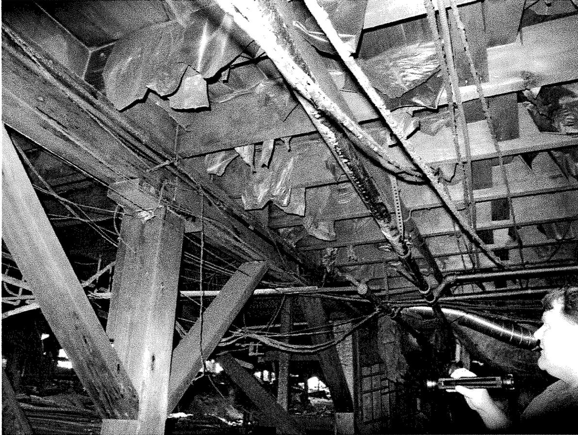
Walking through the basement, it was clear that the fire had spread horizontally in the workshop/crawlspace. Some of the floor joists were burned through, while others were substantially blackened and charcoaled. Under floor wiring had melted away and underfloor duct systems were either burned or collapsed after supports burned through.
